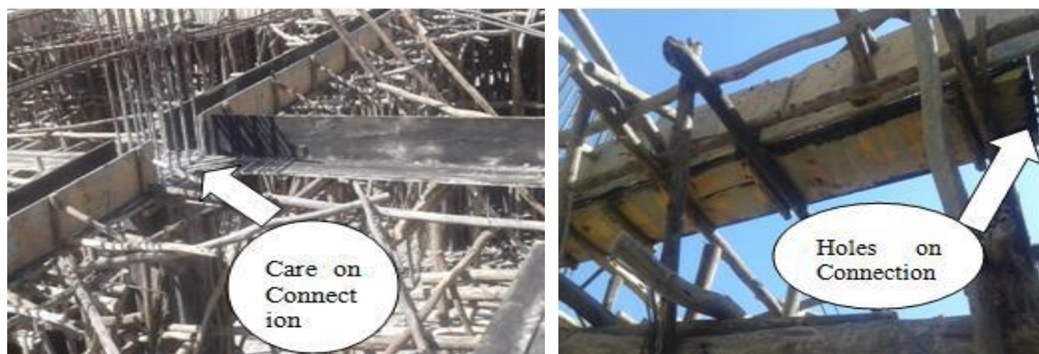
Figure 7. Beam Formwork.
