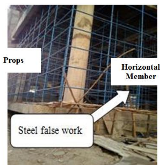
Figure 98. Steel Props.
